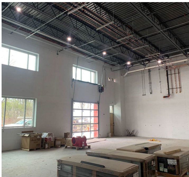
Plumbing and conduit installation in the tech ed suite.
