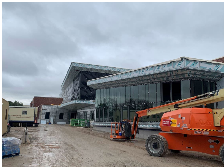
Curtain wall glazing and metal flashing installation is continuing on the south side of the building.
