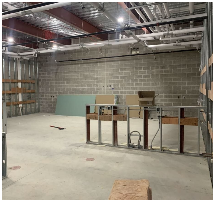
Rough-in work is being done in the culinary lab.
