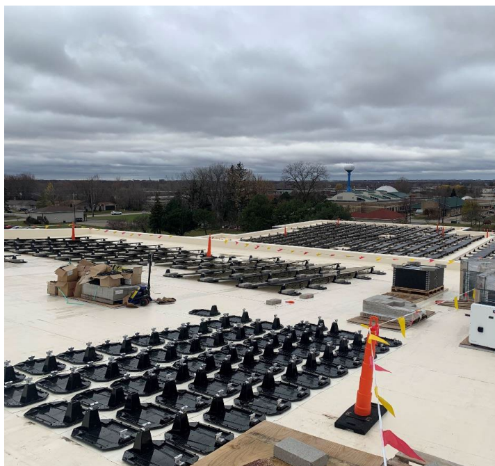
Installation of the rooftop solar array.
