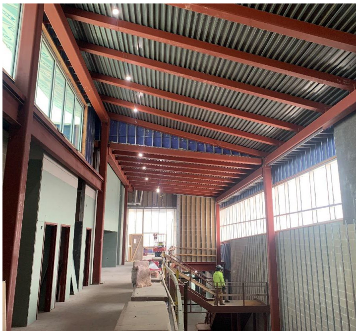
Metal stud framing install at the LMC entry is in progress.
