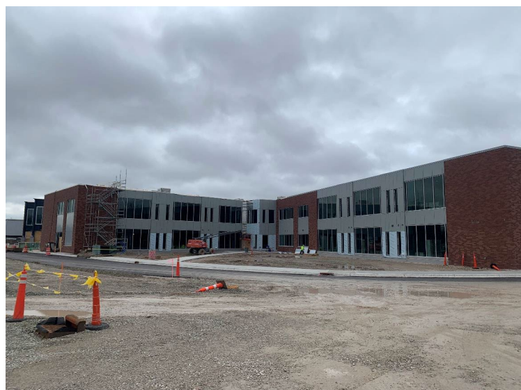
Composite wall panel installation is nearing completion, and exterior electrical devices are beginning to be placed.
